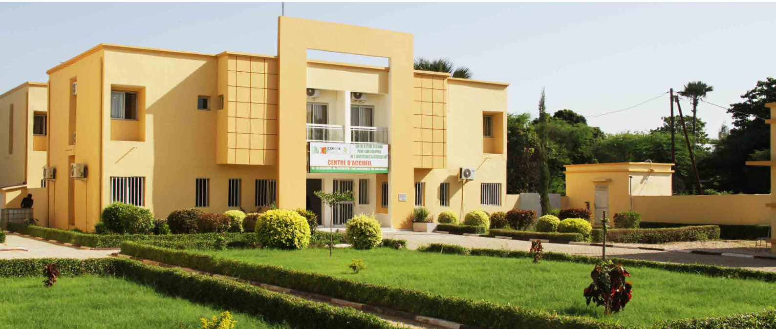
One of the new buildings of the dry cereals Regional Center of Excellence, Thiès, Senegal
