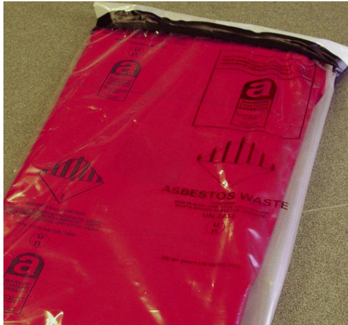
Figure 17: Possible wrapping of asbestos roof sheets after removal
